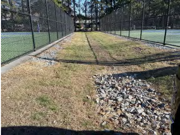
Photo 31: Drainage swale between tennis courts.
