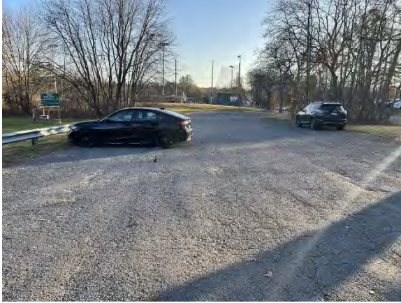
Photo 13: Existing parking lot, lack of discrete spaces/lanes and uneven surface.
