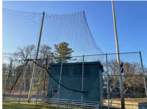
Photo 16: Ball safety netting in poor condition.
