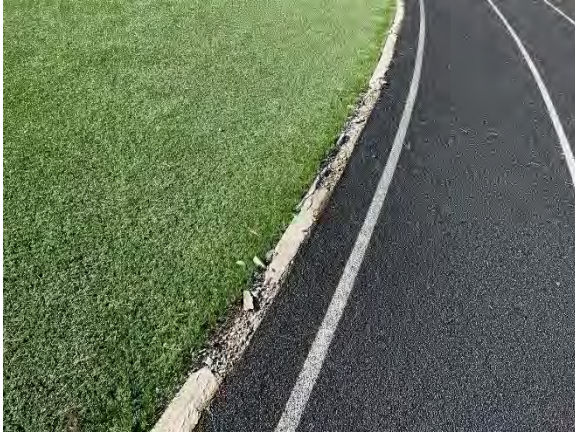
Photo 19: Cracking of anchor curb along the track.
