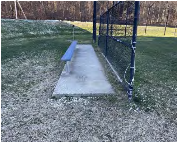
Photo 11: Player benches in good condition but concrete pad uneven with the playing surface.
