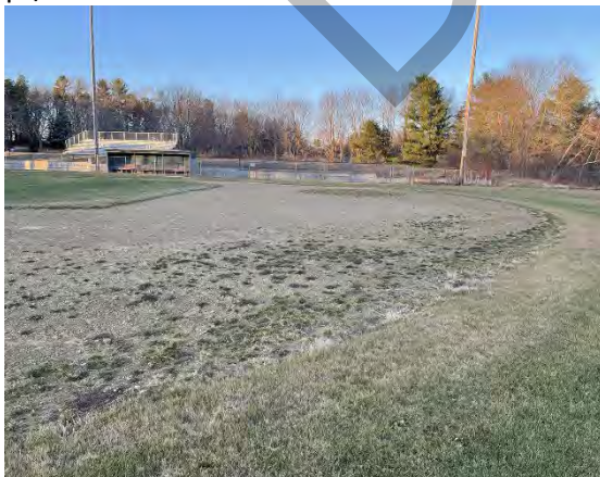
Photo 25: Grass and weed intrusion through infield clay.
