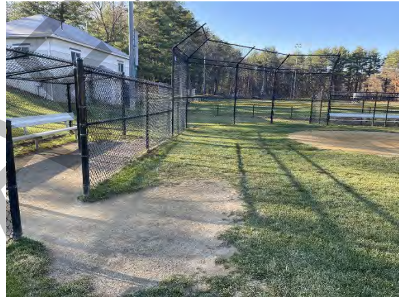
Photo 16: Existing dugout with overused entrance surface. Fencing and backstop in overall good condition.
