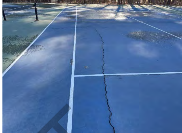
Photo 46: Cracking throughout the court surface.
