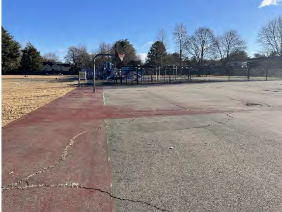
Photo 1: Cracks seen throughout the court playing surface.
