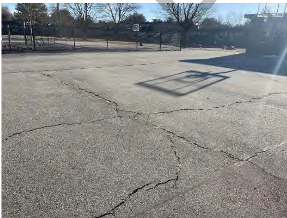
Photo 5: Cracking and fading of the court surfacing.
