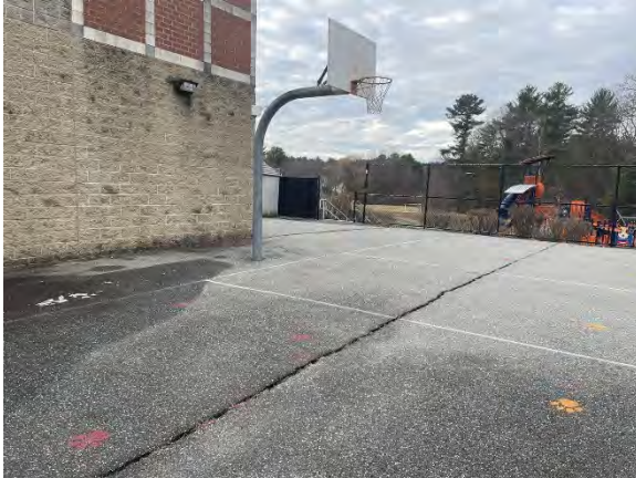
Photo 1: Cracking through the court surface.
