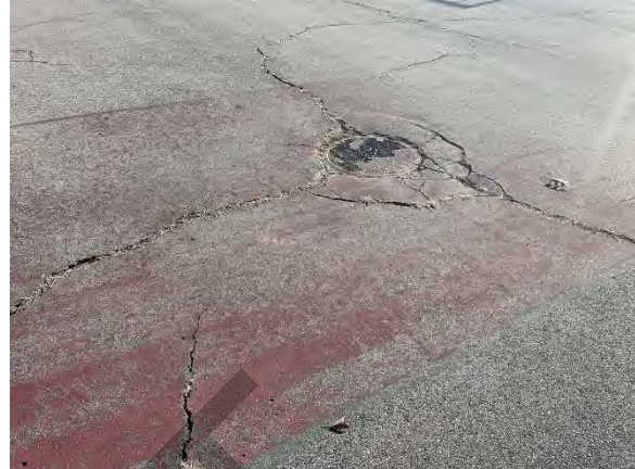
Photo 2: Cracks and divot at the drain manhole.
