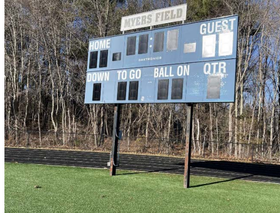
Photo 20: Scoreboard in fair condition with some rusting.
