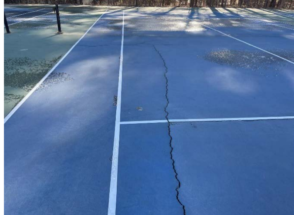
Photo 46: Cracking throughout the court surface.
