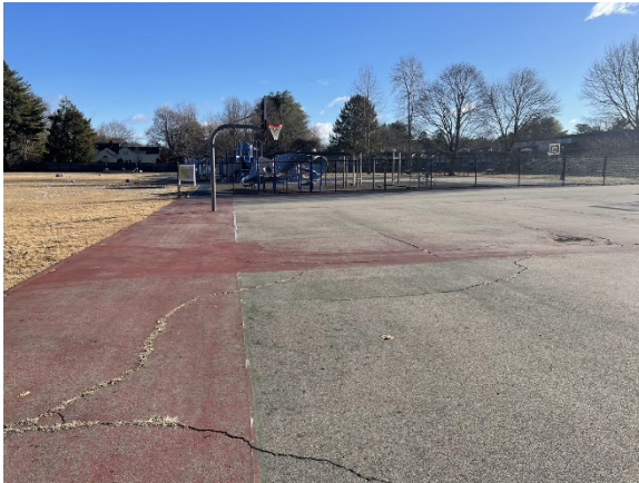
Photo 1: Cracks seen throughout the court playing surface.
