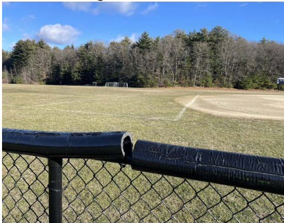
Photo 3: Soccer field striping overlapping clay infield. Fencing safety cap in poor condition.
