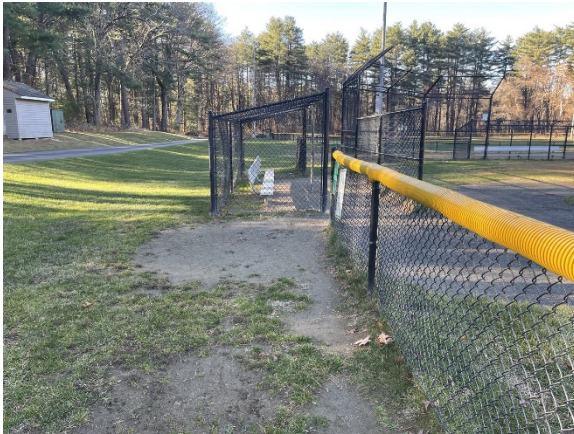
Photo 19: Fencing in overall good condition with yellow safety cap. Overused entrance surface.
