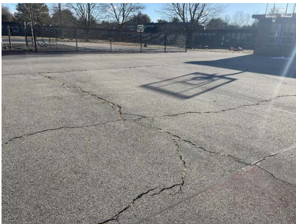
Photo 5: Cracking and fading of the court surfacing.
