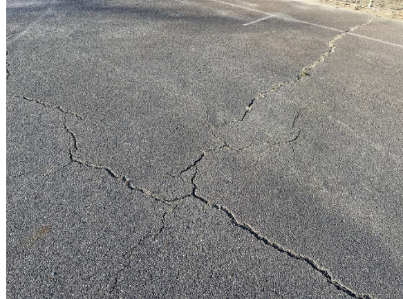
Photo 2: Minor cracking throughout the surface.
