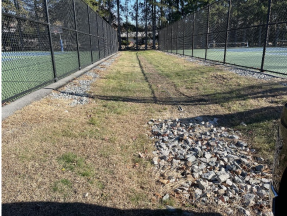
Photo 31: Drainage swale between tennis courts.
