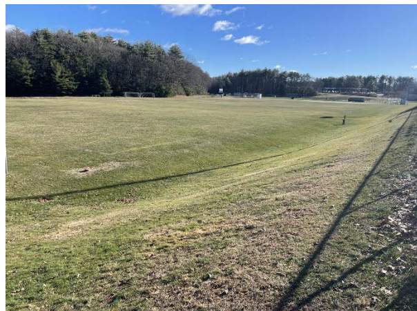
Photo 18: Swale between the stadium field and practice fields.
