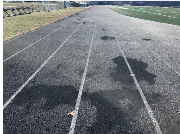
Photo 28: Overused patches throughout the track surface.
