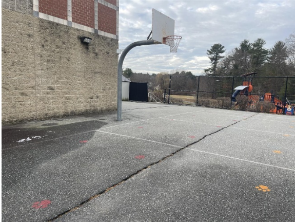
Photo 1: Cracking through the court surface.
