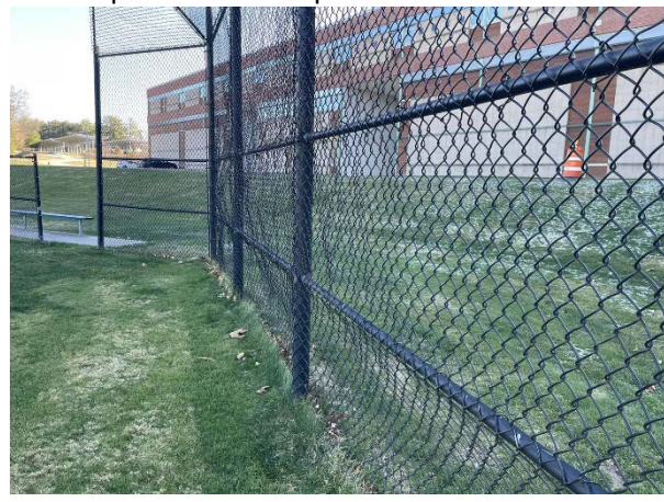
Photo 12: Backstop in fair condition with some bowing of the fence.
