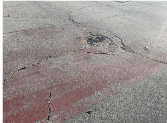
Photo 2: Cracks and divot at the drain manhole.
