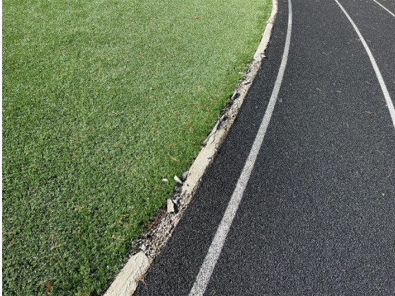
Photo 19: Cracking of anchor curb along the track.
