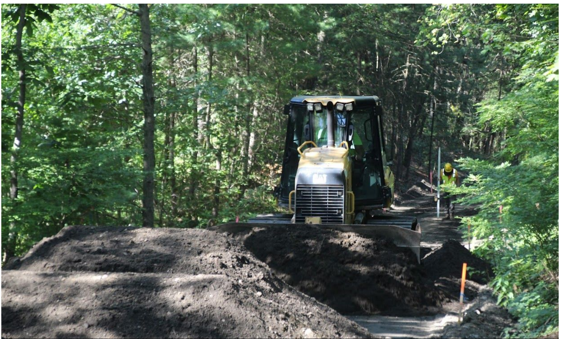
August 23, 2023: Leveling and grading of subsurface material at Old Lancaster Rd 66
