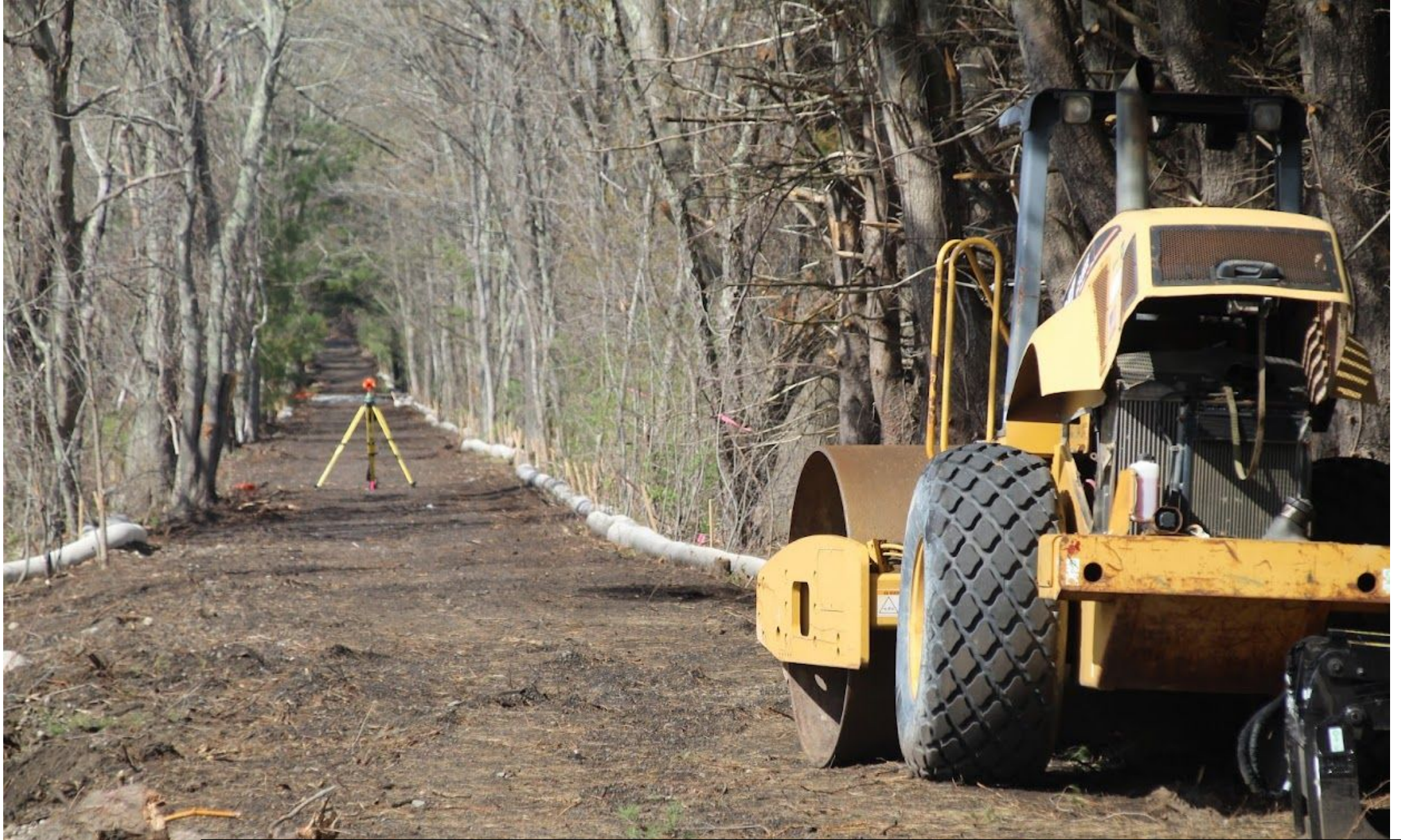
April 24, 2023: Surveying and leveling the corridor north of Codger Lane.
