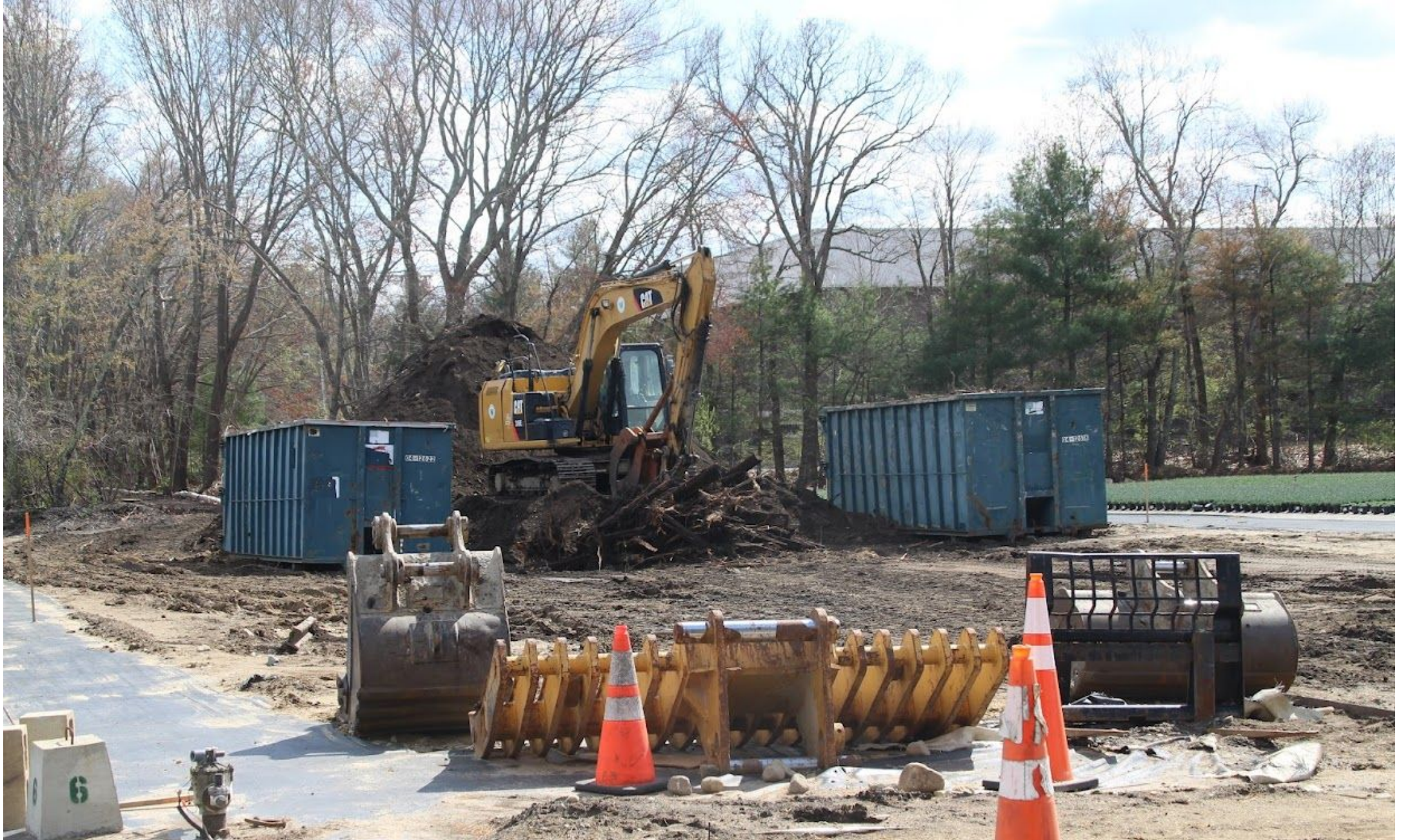
April 24, 2023: Tie removal, preparing the rail trail corridor south of Codger Lane.
