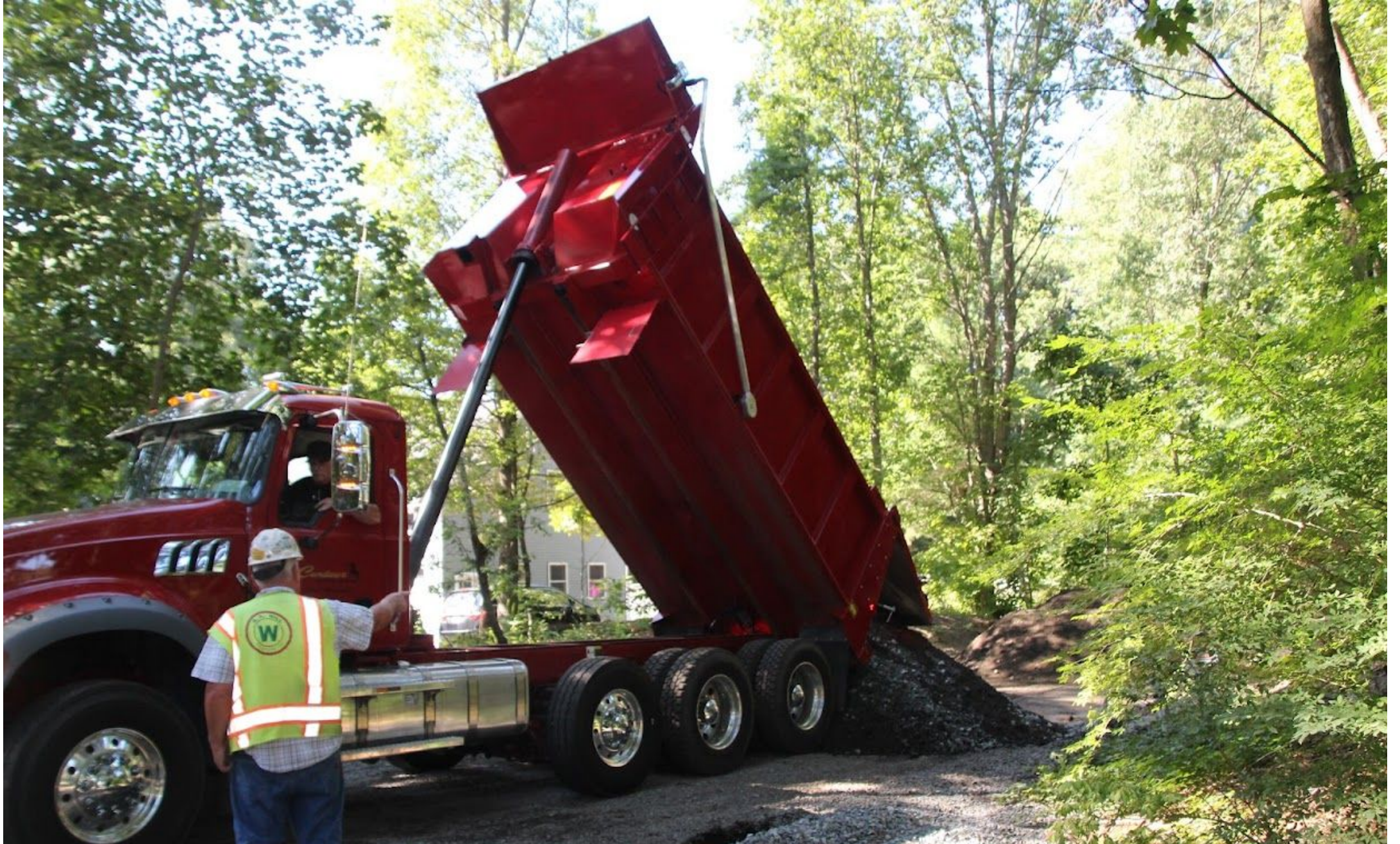
August 23, 2023: Subsurface material delivery at Old Lancaster Rd.
