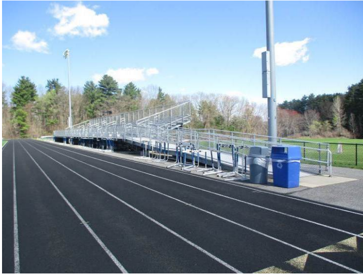
The durable steel-framed, aluminum spectator bleachers remain in good current condition.
