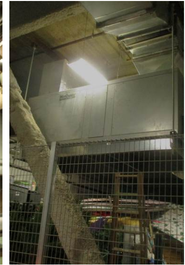
The lower-level automotive shop and the baseball batting cage room are heated and ventilated by individual ceiling-mounted, hydronic heating/ventilation units (HV-1 and HV-2) that are connected to the boiler-water loop.
