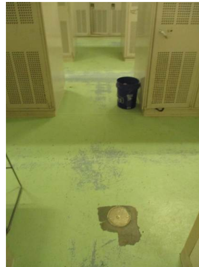
Age and hard-use related flooring wear and locker damage observed at the boys locker room.
