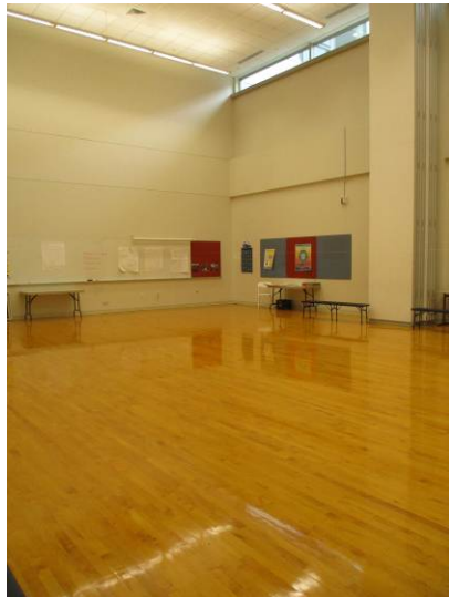
The wood-strip flooring at the Multi-Purpose Room also undergoes an annual buff and coat refinishing cycle and remains in good current condition.
