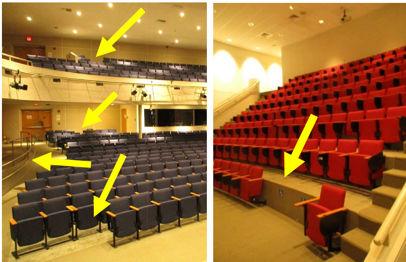
The auditorium and lecture hall feature compliant wheelchair spaces at both levels; and access routes and ramps to those spaces with compliant dual-height continuous handrails.
