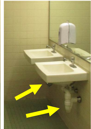
A similar issue exists at the multi-stall hallway restrooms. One sink features covered piping, the other does not.
