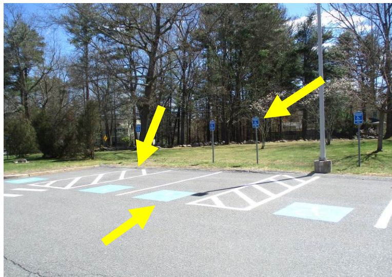
The accessible parking stalls at the front/main entrance parking lot feature compliant access-aisles, surface symbols, and standing designation signs.
