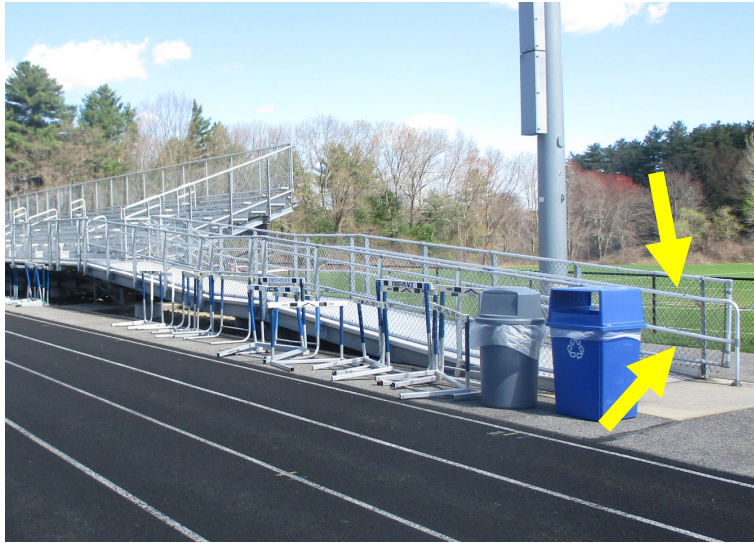
The stadium bleachers feature a compliant access ramp with dual-height continuous (uninterrupted) handrails.
