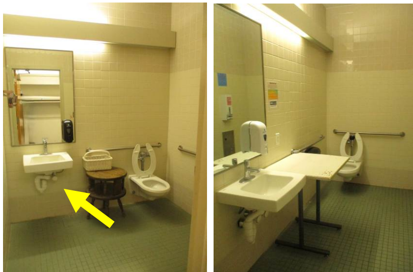
The barrier-free accessible hallway and locker-room single-user restrooms feature compliant sink and mirror heights; toilet and grab-bar positioning; and covered/insulated under-sink piping.
