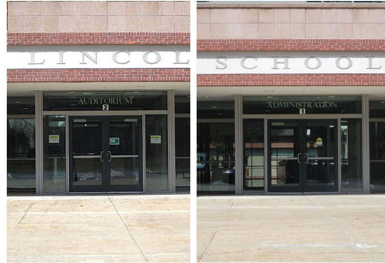
The auditorium and admin entrances feature standard-size commercial wide-stile aluminum and glass entry doors that remain in good current condition (no issues reported).
