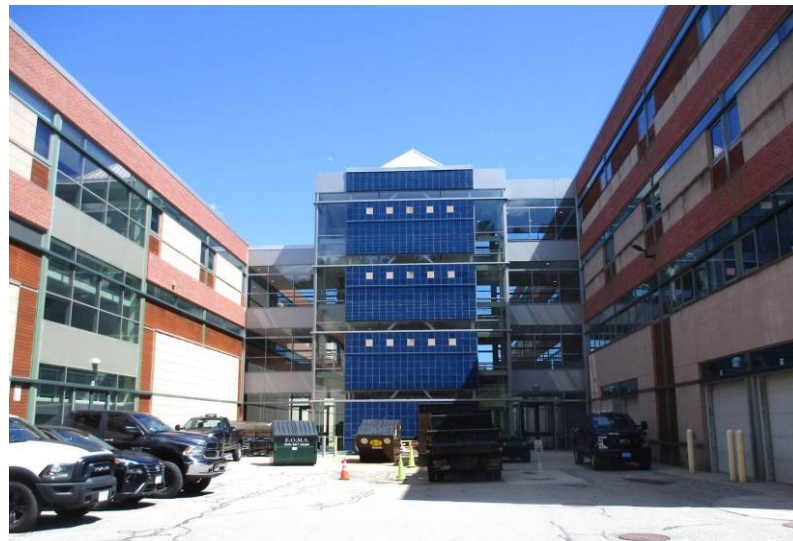
Typical building architecture observed at the upper (A-B) and lower (B-C) west-facing maintenance/service courtyards.
