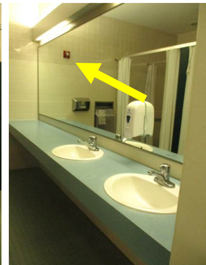
All restrooms and locker-rooms feature compliant audio-visual horn/strobe fire alarm warning devices.
