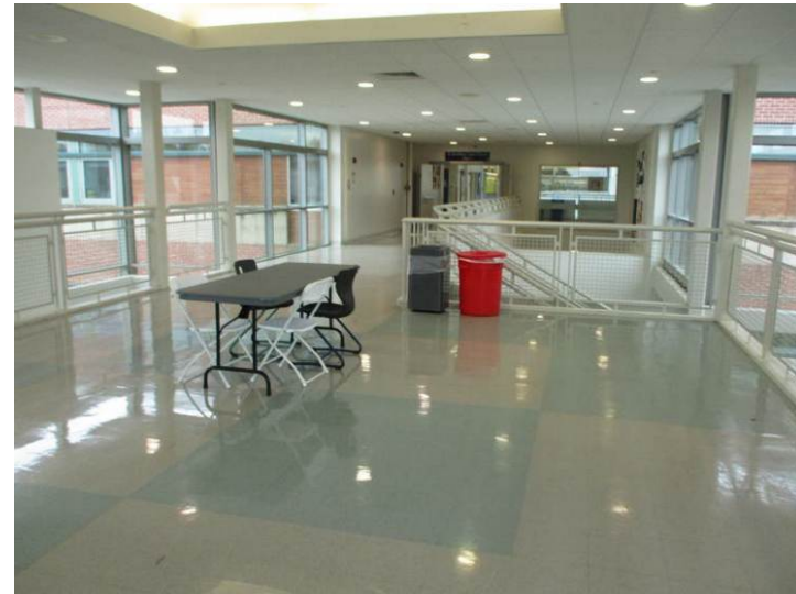
Typical connecting corridor finishes and conditions. The vinyl tile flooring is stripped and polished annually (every summer) and buffed regularly throughout the school year.
