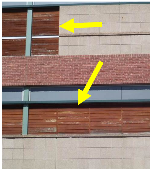
The horizontal and vertical stained-wood cladding is in need of near-term re-staining/sealing and possible eventual replacement with a more durable and low-maintenance composite-material cladding.
