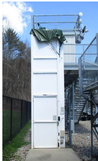
The raised announcer's booth and enclosed National Wheel-O-Vator, 750-pound-capacity accessible platform lift (at the west side of the field) were both newly installed circa 2010.
