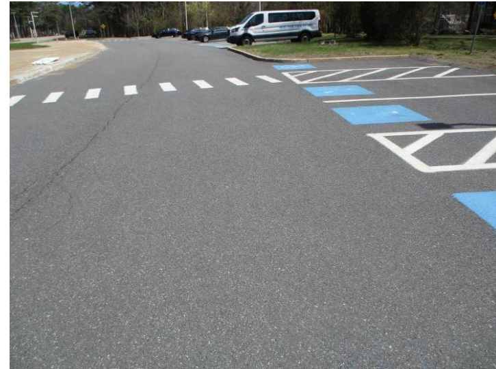
The front/main-entrance parking lot was resurfaced in 2020 and remains in good current condition.
