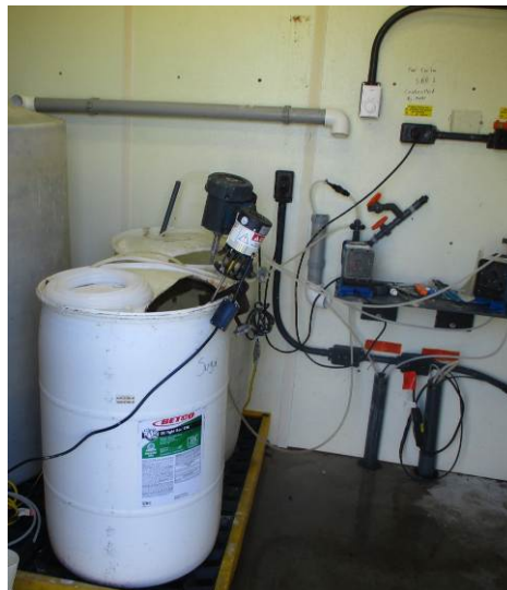
The small facility building contains the system control panels and automatic feed system tanks and controllers.
