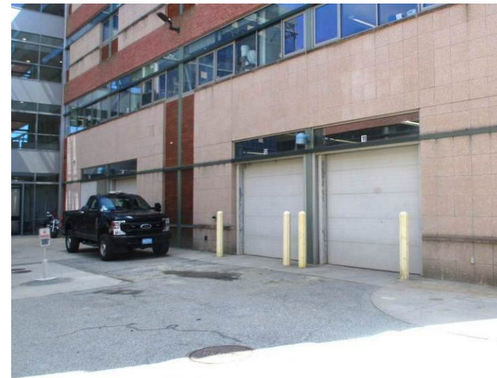
The lower (B-C) service courtyard features the auto shop and shipping/receiving bays with three large commercial segmented-panel overhead garage doors.
