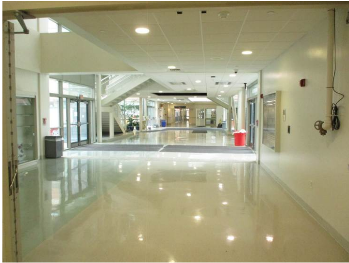
The lower-level connector finishes (between the B and C sections) and four of the problematic large oversized double-leaf front and rear entry doors.
