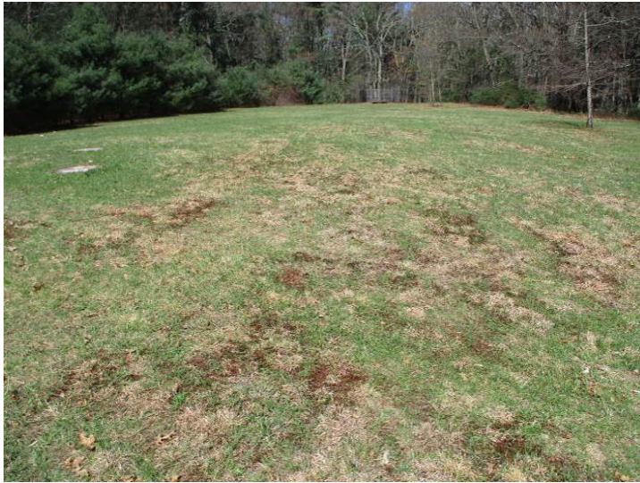
The treated/clarified wastewater is eventually pumped up to a large, raised leaching field located above the facility at the east side of the property.
