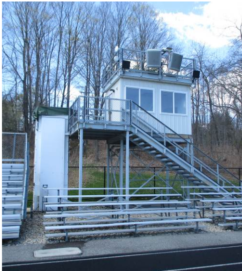
The raised announcer's booth and enclosed National Wheel-O-Vator, 750-pound-capacity accessible platform lift (at the west side of the field) were both newly installed circa 2010.
