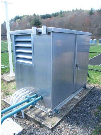
The commercial irrigation system features a Flowtronex packaged pumping system, two commercial Rain-Master Eagle timer/control panels, and two submerged irrigation well pumps.
