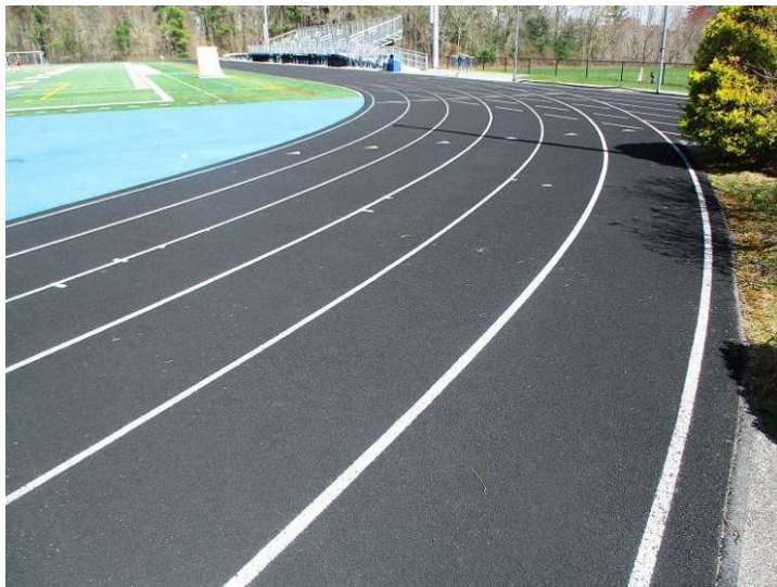
The rubberized running track and stadium field D-area were originally installed in 2007, and a subsequent structural spray resurfacing was completed in 2019.
