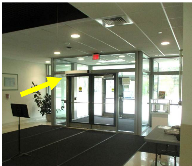
The front/main entrance vestibule features accessible power-assist openers at the exterior and interior doors.
