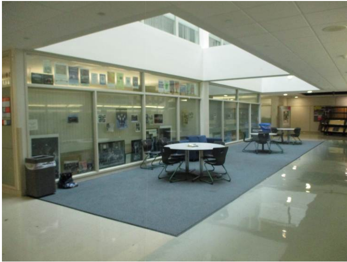
Various corridor lounge/study/gathering areas feature broadloom carpet flooring that reportedly dates to the original 2004 construction.
