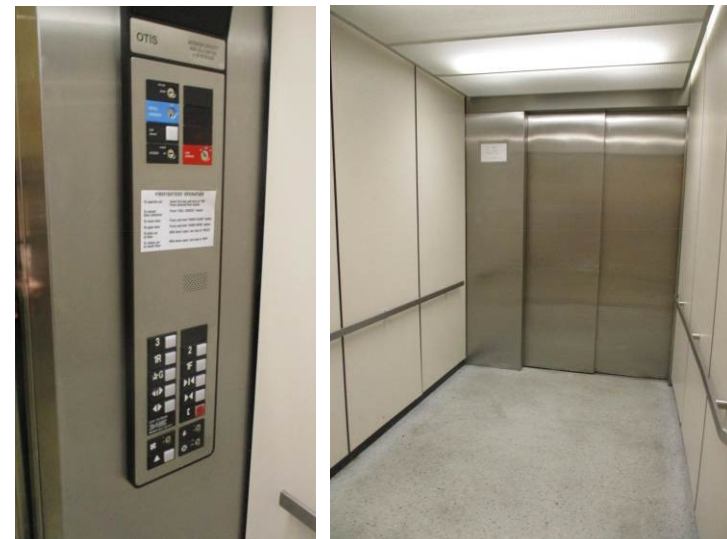
The B-section elevator cab finishes, door/floor buttons, and dual (front and rear) access doors.
