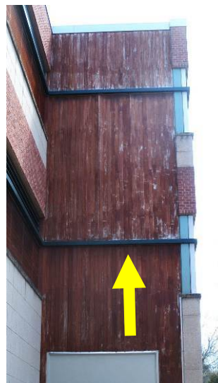
The horizontal and vertical stained-wood cladding is in need of near-term re-staining/sealing and possible eventual replacement with a more durable and low-maintenance composite-material cladding.
