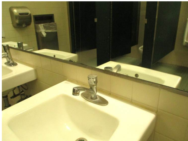
All single-user and multi-stall restroom and locker-room sinks feature push-style faucets which is ADA acceptable.
