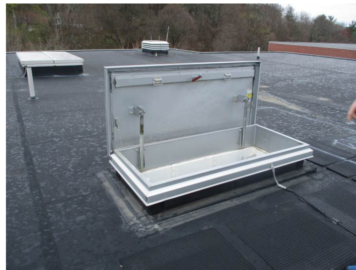
Sections A and B feature large galvanized-steel roof access hatches. The Section C roof is access from a doorway at the north connector/stair-tower.
