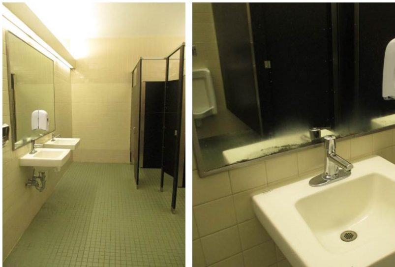
Typical finishes, fixtures, and visible age and use-related wear observed at the various boys and girls multi-stall restrooms.
