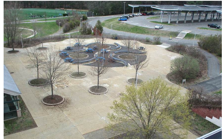
The cafeteria plaza features a mix of concrete and asphalt flatwork, painted-metal serpentine benches and picnic tables, and pole-mounted LED surface lighting fixtures.
