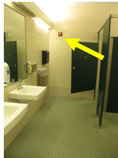
All restrooms and locker-rooms feature compliant audio-visual horn/strobe fire alarm warning devices.
