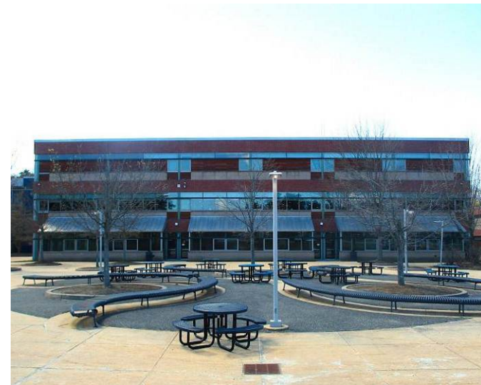
The east-facing elevation of the B section features the ground-floor cafeteria and two sets of standard-size, double-leaf, aluminum and glass plaza doors.
