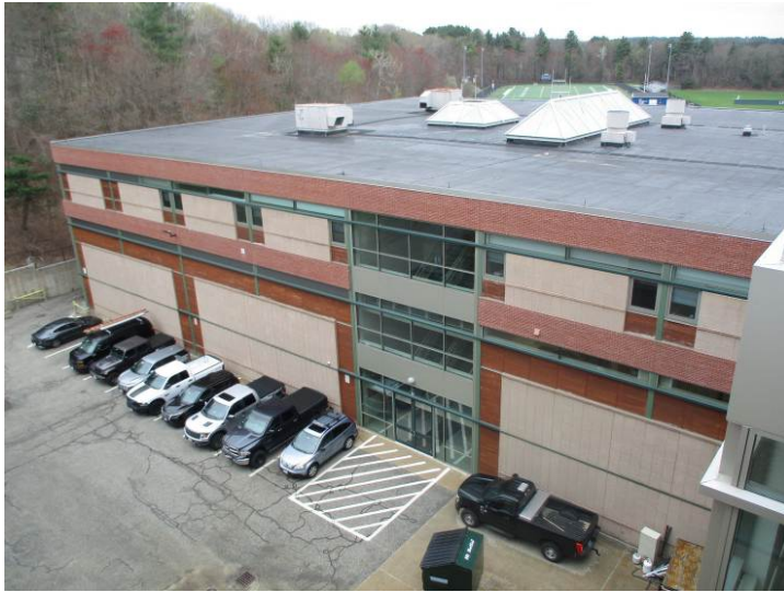
The south-facing elevation of Section C at the east-facing (rear) lower service courtyard.
