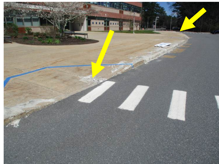
The access routes between the accessible parking stalls and the various front-elevation entrance and egress doors feature compliant curb-cuts.
