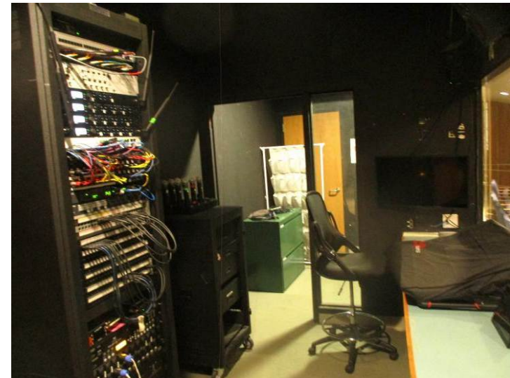
The ageing, outdated, lighting systems at the Auditorium, Black Box theatre, and Lecture Hall are all reportedly in need of a full overhaul/upgrade/replacement. The sound systems were recently updated in 2025.
