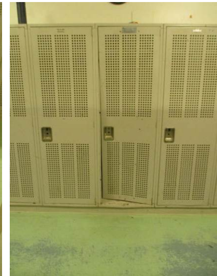
Age and hard-use related flooring wear and locker damage observed at the boys locker room.
