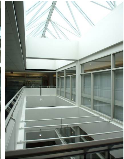
Typical steel-framed aluminum and glass curtain-wall assemblies (at the connecting corridors), and multi-level open courtyards illuminated by large aluminum and glass skylight assemblies.
