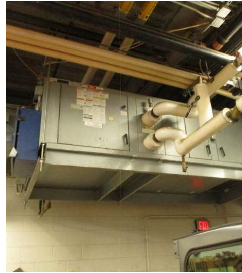
The lower-level automotive shop and the baseball batting cage room are heated and ventilated by individual ceiling-mounted, hydronic heating/ventilation units (HV-1 and HV-2) that are connected to the boiler-water loop.
