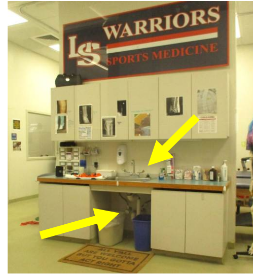
The Sports Medicine room cabinetry features a compliant roll-under sink with covered under-sink piping (to protect against potential roll-under knee-impact injury) and a compliant lever-style faucet.
