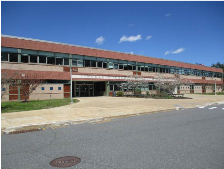
The south-facing (front) elevation of the A-section. This section features two above-grade levels, one below-grade level, and the auditorium and administration entrances.
