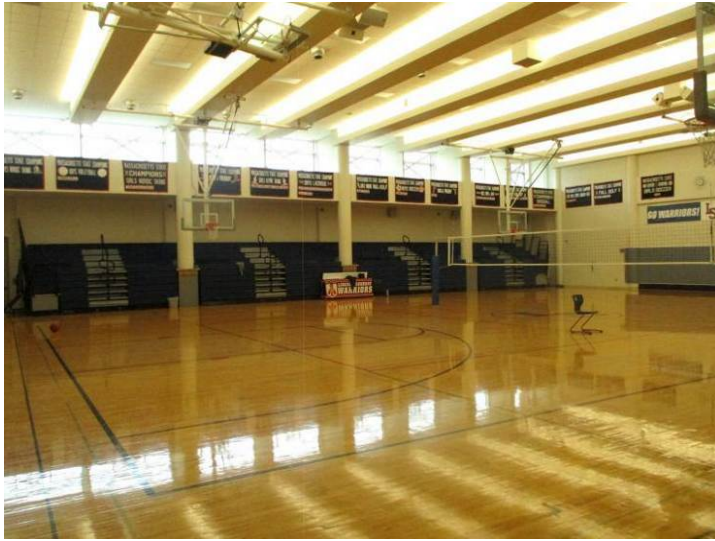
Gym 1 features a finished wood-strip flooring. A buff and coat (screen and re-coat) maintenance refinishing cycle is completed annually (per management).
