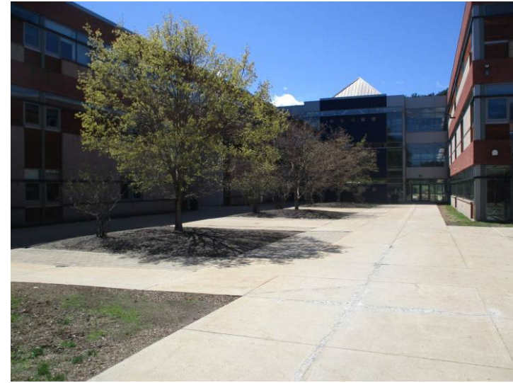
The east-facing upper (A-B) courtyard features the student entrance with standard-size double-leaf commercial aluminum and glass entry doors.
