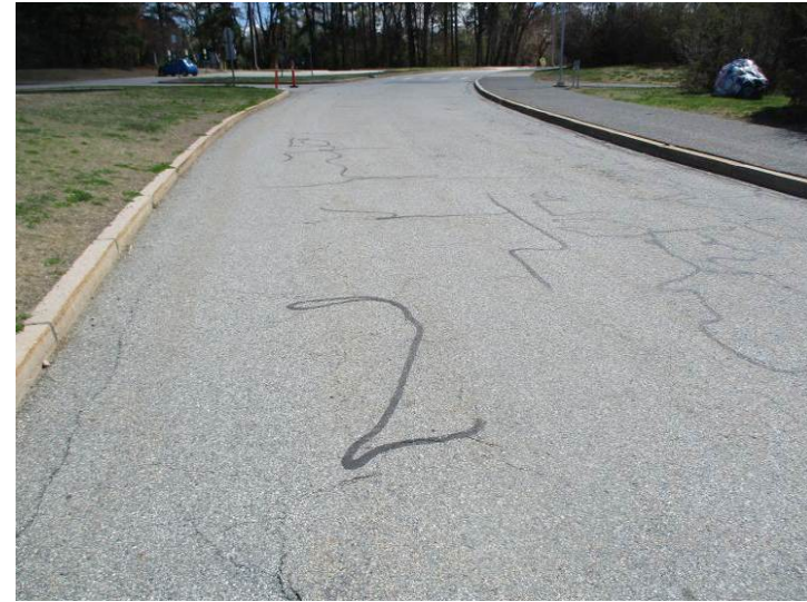
Typical roadway asphalt surface conditions.
