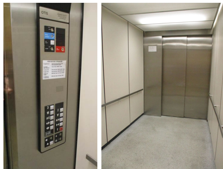
The elevator cabs feature compliant maneuvering room and door/floor buttons positioned at compliant height.
