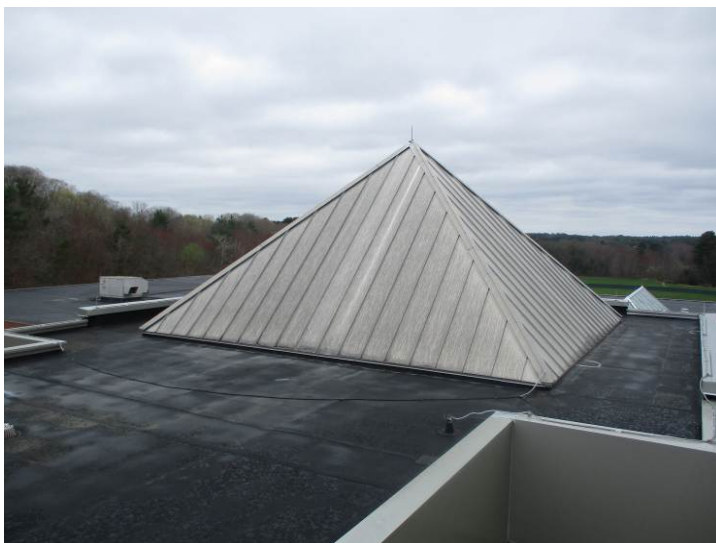
The two connecting corridor/stair-towers feature decorative architectural pyramid structures with durable standing-seam metal roof coverings.
