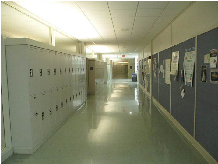
Typical corridor finishes and student lockers. A new building-wide digital interior lighting control system was installed in 2025; however, installation-related operating issues and contractor trouble-shooting is still ongoing.
