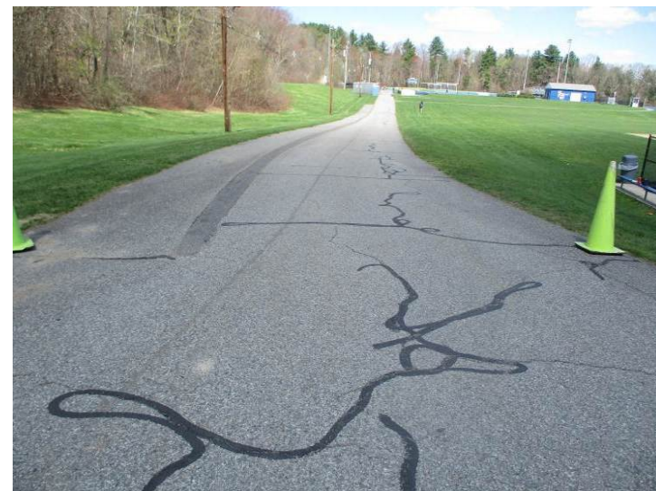
The stadium roadway and adjacent walkway conditions.
